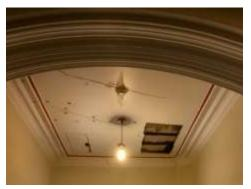
when the ceilings in the hallway were inspected, serious issues were identified. A considerable amount of historic water ingress had occurred, and some joists had substantially rotted. Fortunately, the damage had only occurred in two sections of the ceiling and Keith's team were able to save most of the fine ceiling architrave and central ceiling rose. Where the architrave could not be saved,
