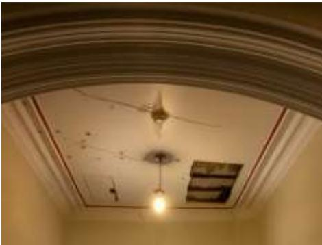
when the ceilings in the hallway were inspected, serious issues were identified. A considerable amount of historic water ingress had occurred, and some joists had substantially rotted. Fortunately, the damage had only occurred in two sections of the ceiling and Keith's team were able to save most of the fine ceiling architrave and central ceiling rose. Where the architrave could not be saved,
